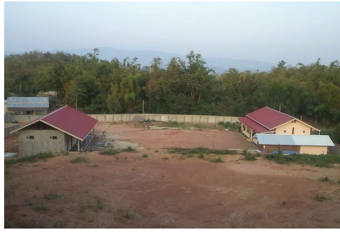
Progress on our Burma property
