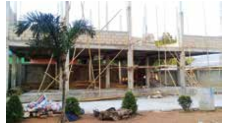
Skills and office building construction.
