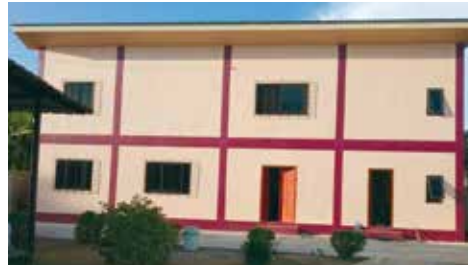
Completed Skills Center building.
